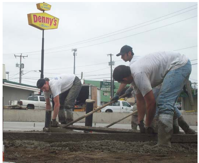
The crew smooths the concrete of the new building floor.
