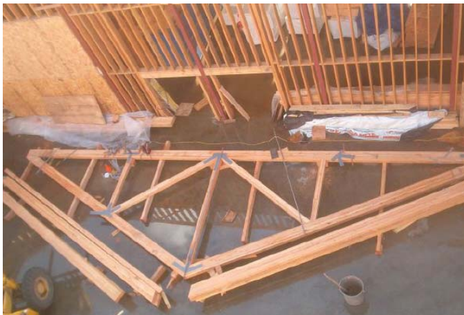
Construction of one of the main roof trusses
