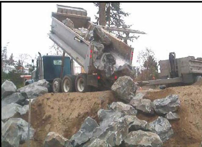
*One load of boulders delivered for the parking lot retaining wall. Each boulder was placed individually by an operator in an excavator.*
